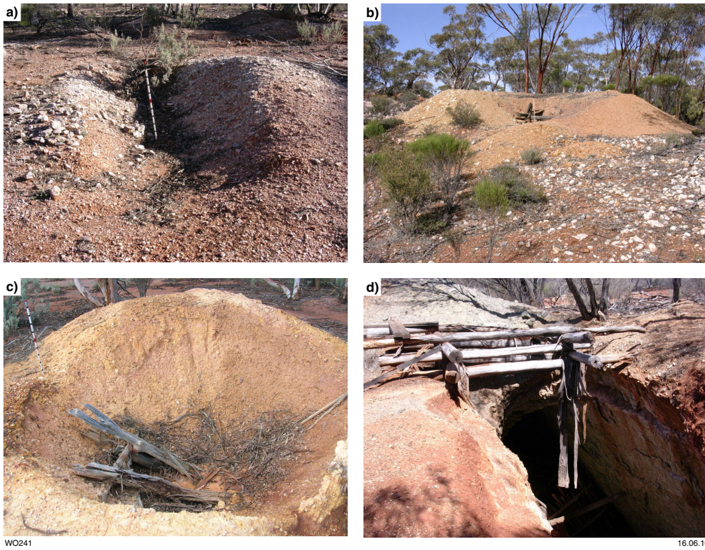
Figure 1.8 Typical examples of bedrock-gold excavations from the abandoned mine sites database: a) shallow working; b) shaft; c) collapsed shaft; d) open stope.
