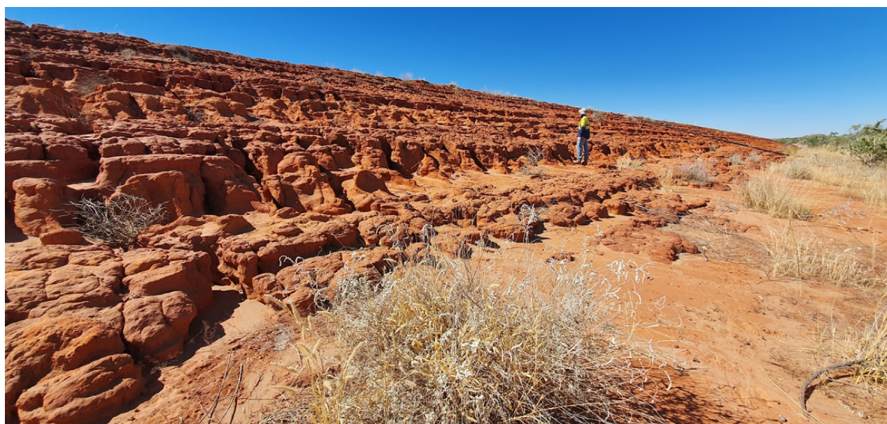
Figure 1. Ellendale 9 TSF-1D Cell 3 western wall, indicating significant gullying and sediment deposition. Gullies are greater than 2 m deep and extend from crest to toe. Remediation options will include rock armouring and modifications to the outer batter slope angle
